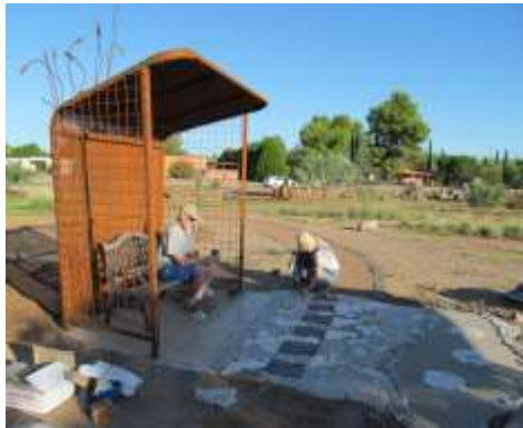
Stacie Meyer and Gary Campbell laying tile mosaic
